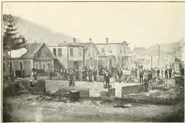
SOUTH ROYALTON AFTER THE FIRST FIRE, FEB. 6, 1878.
